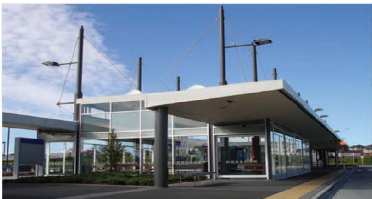
One of the Northern Busway Stations
