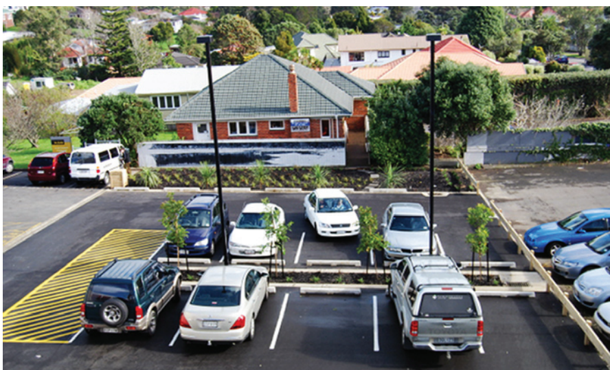
Features outside the building include planting to shade vehicles and a rain garden at the back of the car park with a compost bin.
