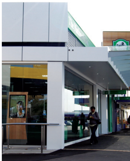
National Bank Blockhouse Bay.
