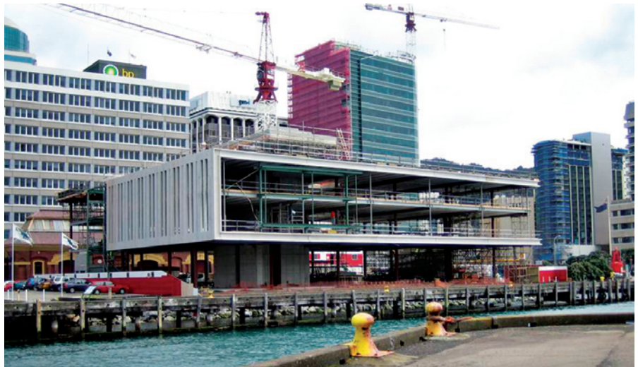
The Meridian Building during construction on the Wellington waterfront.
