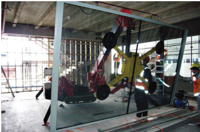
Placing the large glazing units.
