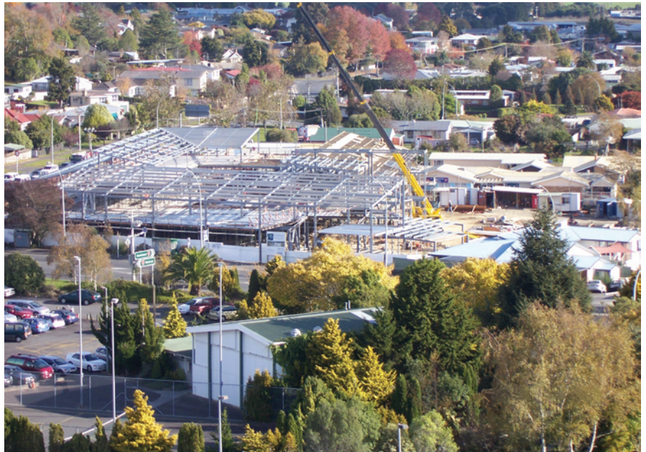
Hamilton's new green hospital during construction.
