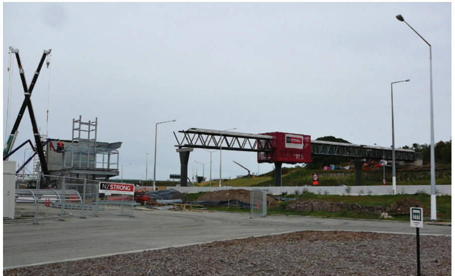
Gantry trolley on 120 m bridge over SH1 Motorway.
