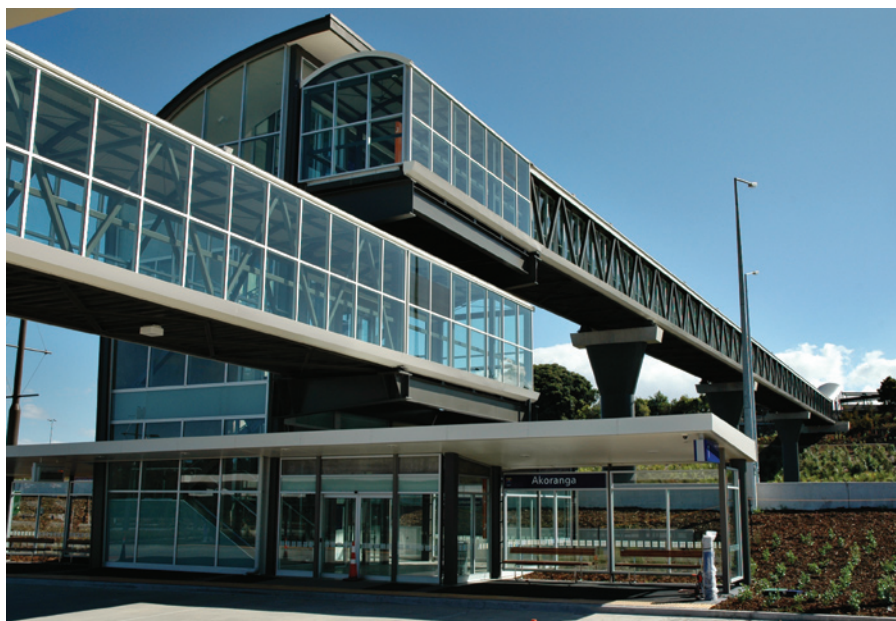
Completed Akoranga Station for the Northern Busway.
